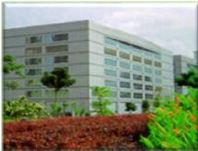
Fuel for Gas District Cooling
