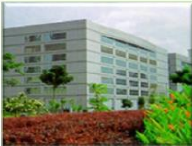
Fuel for Gas District Cooling
