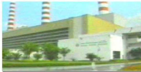
Fuel for Power Generation
