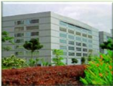
Fuel for Gas District Cooling
