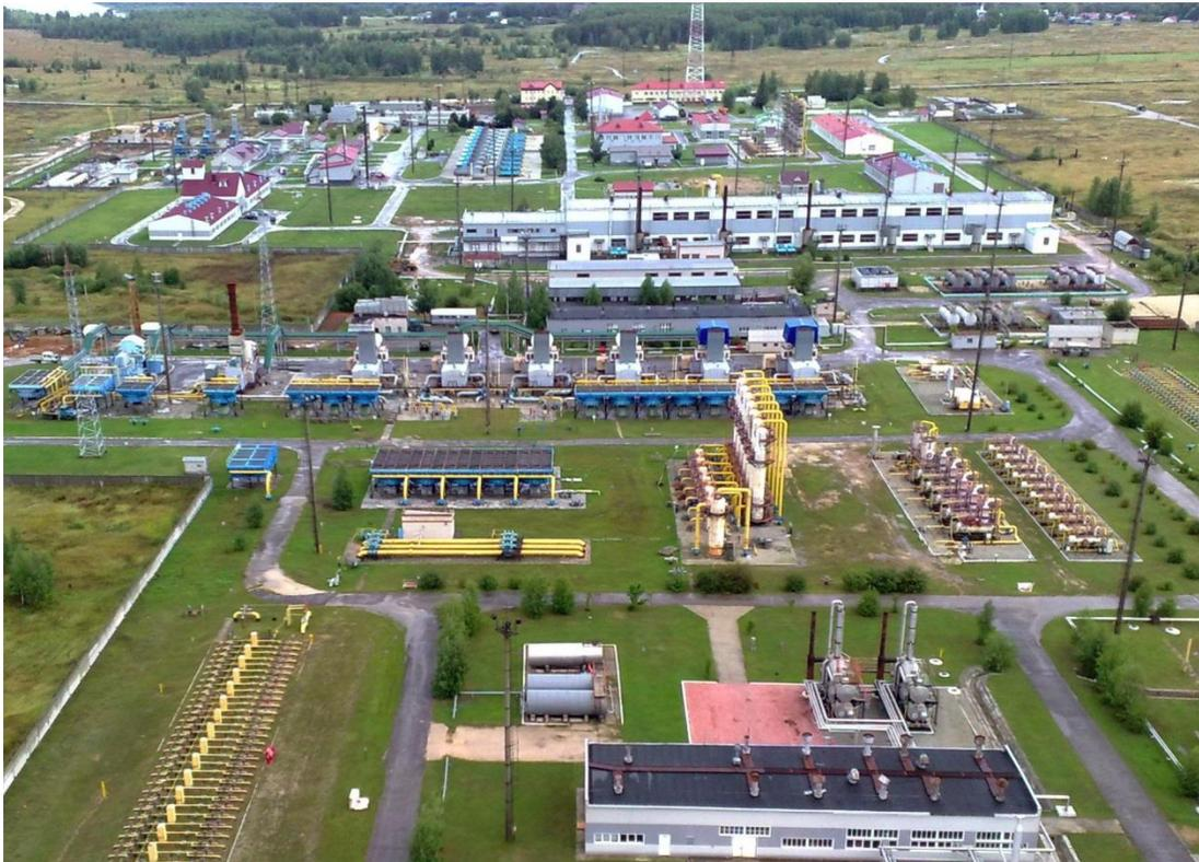
*Fig. 8. Kasimov UGS in the Ryazanskaya region is the world's No. 1 gas storage facility in water-bearing formation (4,5 bcm) (<http://www.gazprom.ru/press/reports/2012/milestones/>).*
