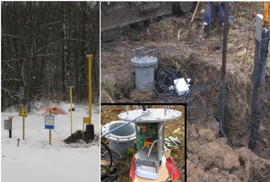
*Fig. 6. System for monitoring pipeline crossings under auto and railroads (SKP21) – underground version.*
