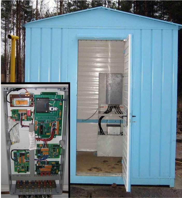
*Fig. 7. System for monitoring pipeline crossings under auto and railroads (SKP21) – above ground container unit.*
